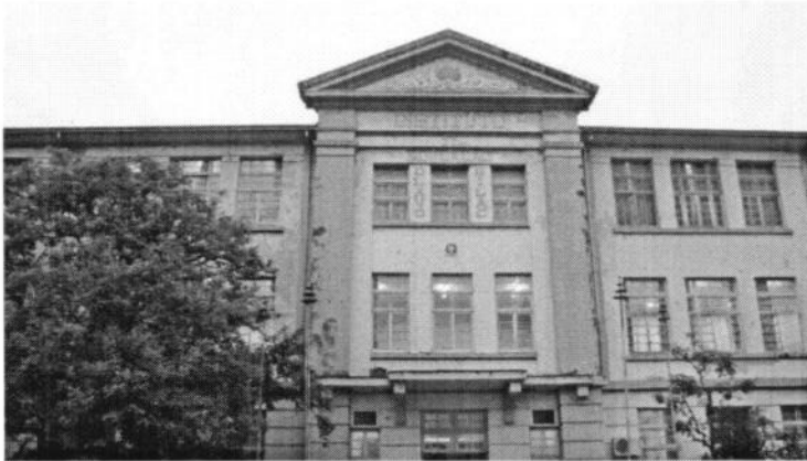
1 Pavilhão Principal - Fachada Principal
