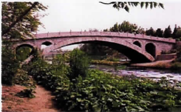
Ponte Zhaozhou, China
