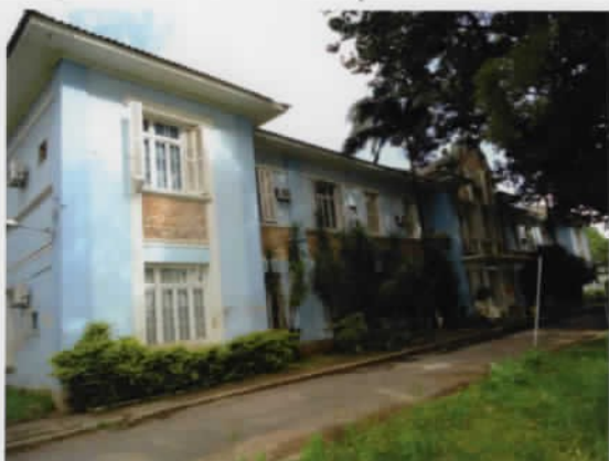
3 Fachada principal - Vista geral
