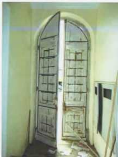
F13. Porta principal - vista interna, 2013.
