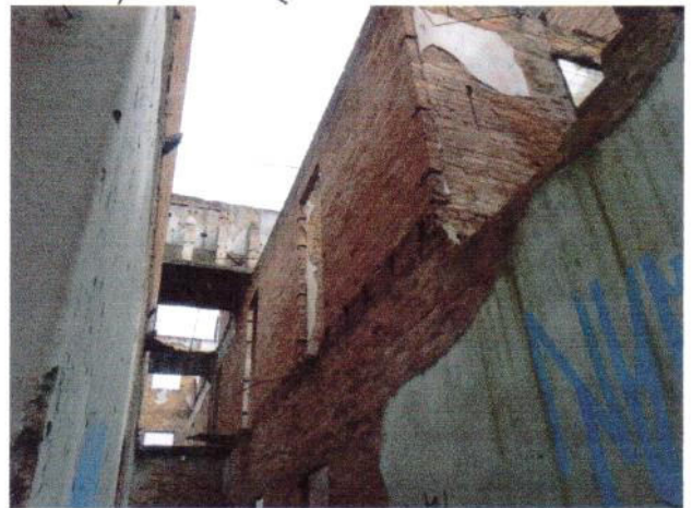
2 Prédio Principal - Corredor central
